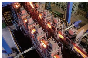
Continuous casting equipment
