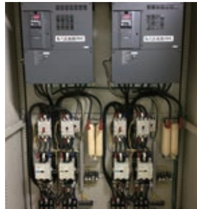
Inverter control panel
