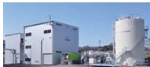
METHASAUROS (Zero-emission sewage sludge reduction, fuel-and fertilizer conversion plant)
