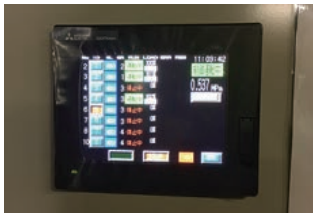
Unit control panel for compressors
