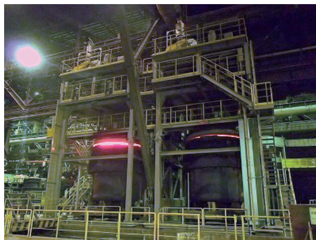
Preheating the ladle
