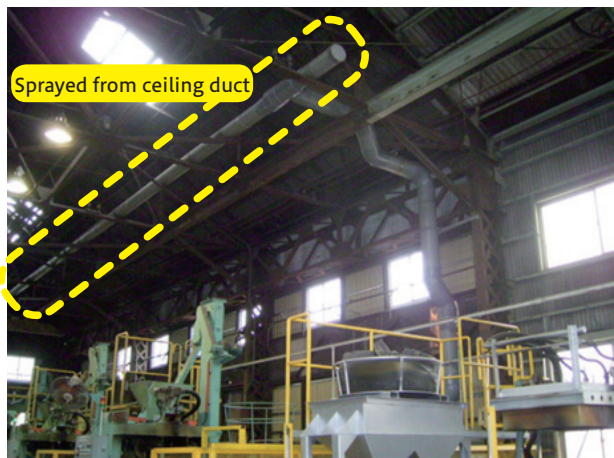
Eliminating odors from the ducts of the mold manufacturing workshop
