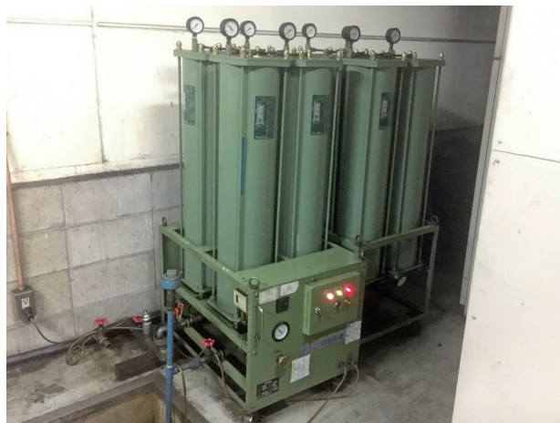
Drain processing equipment
